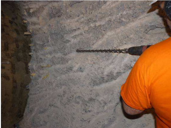
Drilling boreholes for the expansive cement (I)
