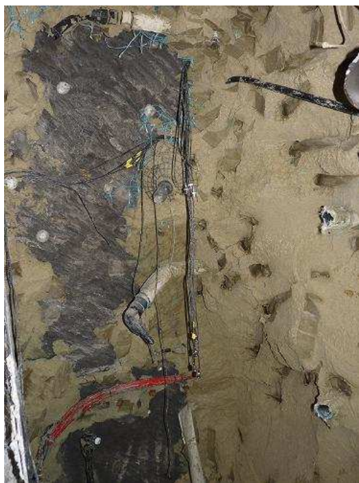
Figure 68: OPA after the dismantling operation
