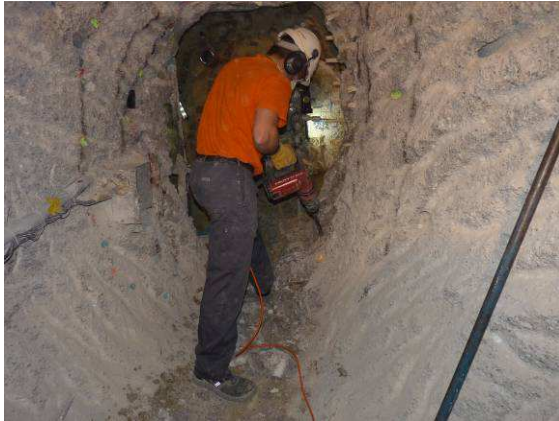
Use of hand tools to remove the concrete plug after the effect of the expansive cement (I)
