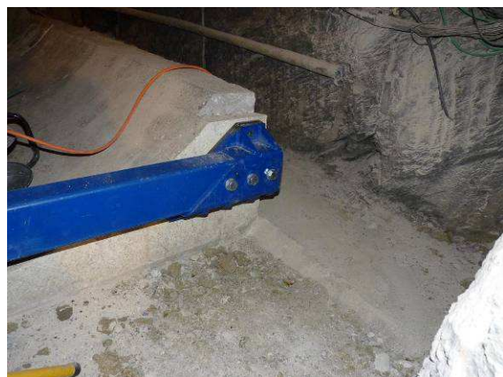
Attachment of the lateral part of the metallic beam to the concrete bed
