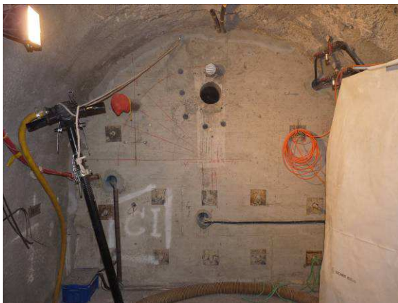
Boreholes around the 200 mm diameter one
