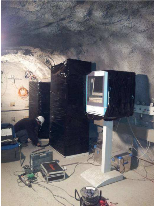
Figure 4: Protection of the cabinets
