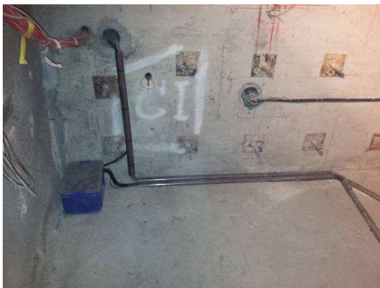
Figure 3: Protection of seismic cables
