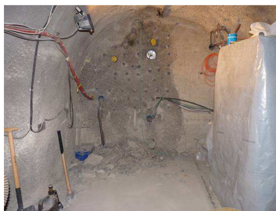
Progress in breaking the concrete of the plug
