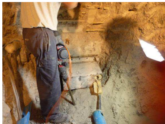
Cable box C dismantling (I)
