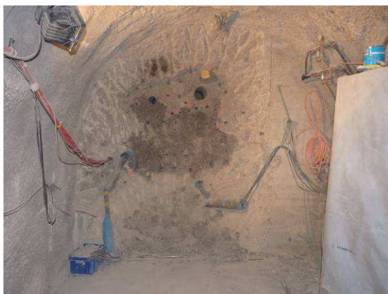
Retaining wall reached
