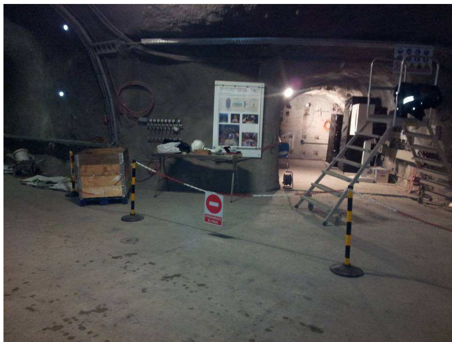
Figure 5: Installation of safety signs
