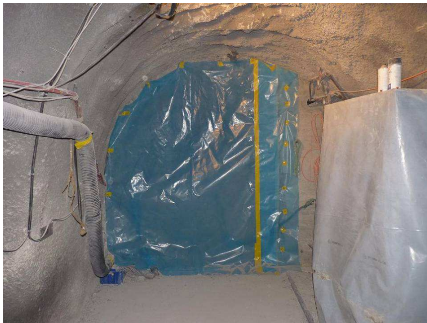
Figure 22: Plastic cover to avoid bentonite drying
