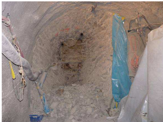
Reaching retaining wall and bentonite
