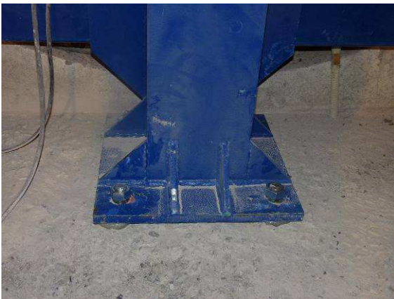
Attachment of the bottom part of the beam to the floor
