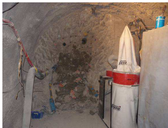
Retaining wall dismantling
