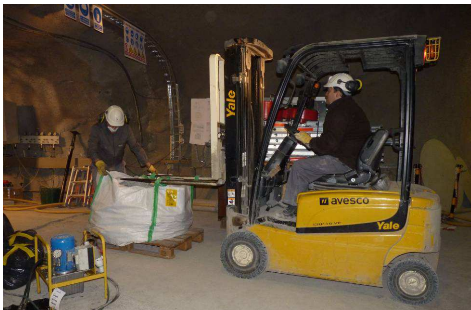
Figure 15: Loading forklift with debris
