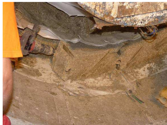
Figure 20: Tools for bentonite blocks removal
