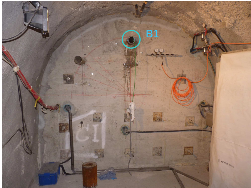
Figure 6: Location of Borehole B1 and planned over coring
