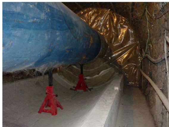
Sawhorses supporting the canister
