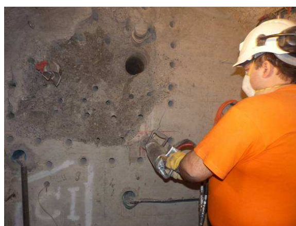
Use of the Darda to break the concrete
