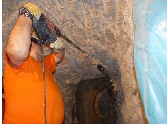
Drilling boreholes for the expansive cement (II)
