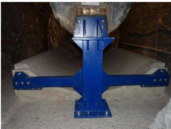
Front view of the metallic beam
