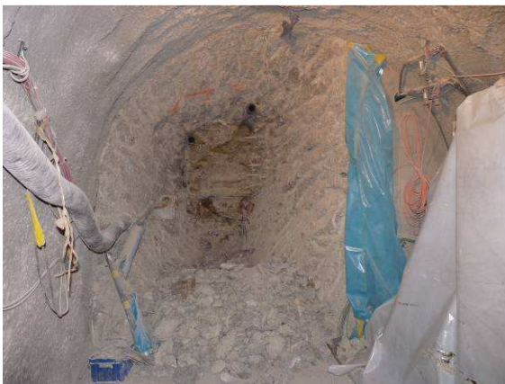
Retaining wall dismantling
