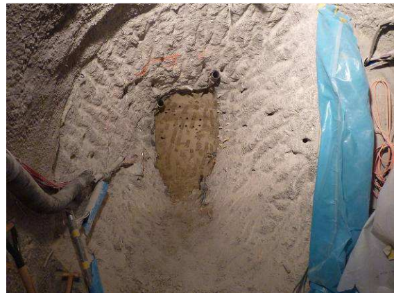
Bentonite in contact with the retaining wall
