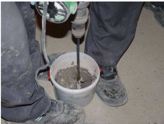
Preparation of the liquid expansive cement
