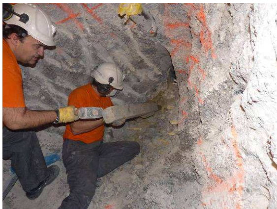
Hammering the sampling pipe into the bentonite
