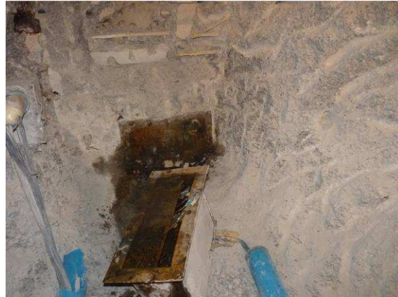
Cable box C dismantling (III). Water spot
