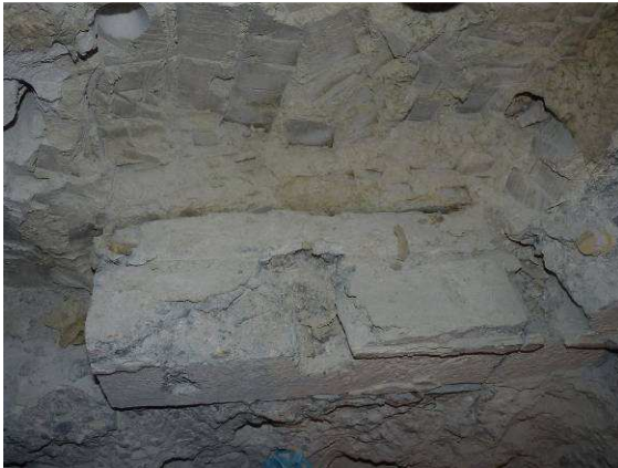
Retaining wall. Concrete/bentonite interface
