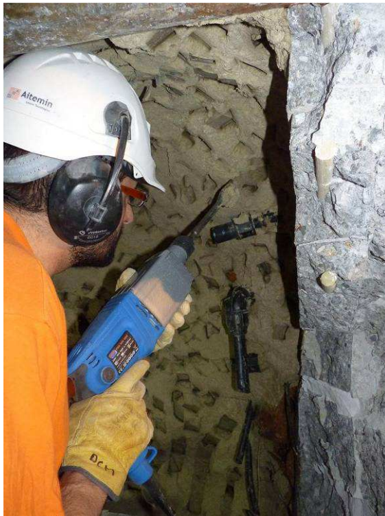
Figure 19: Tools used for bentonite removal
