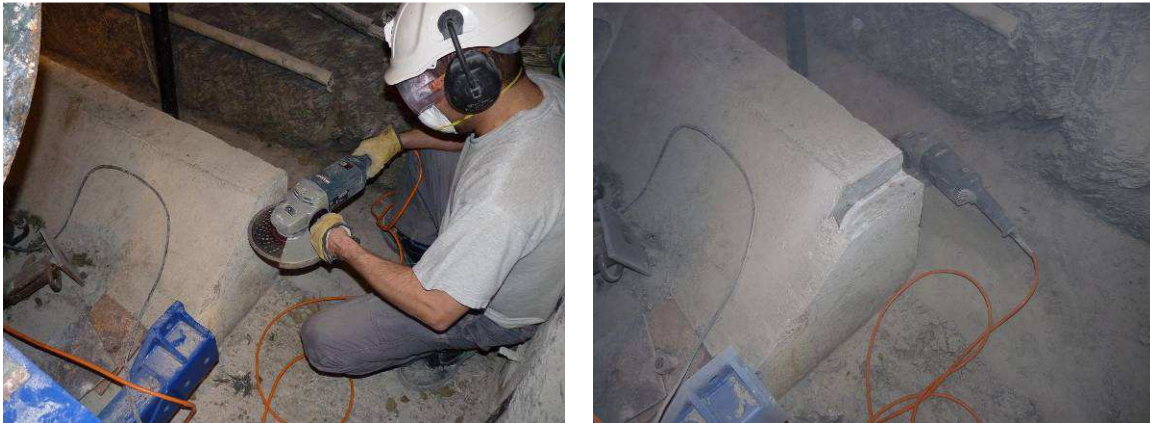
Figure 35: Concrete bed sampling
