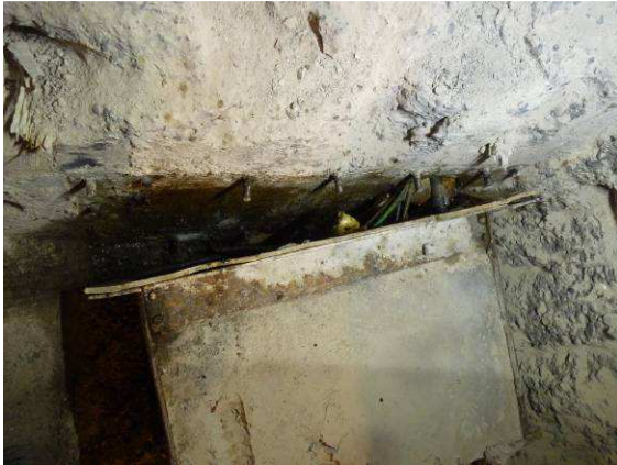
Cable box C dismantling (II)
