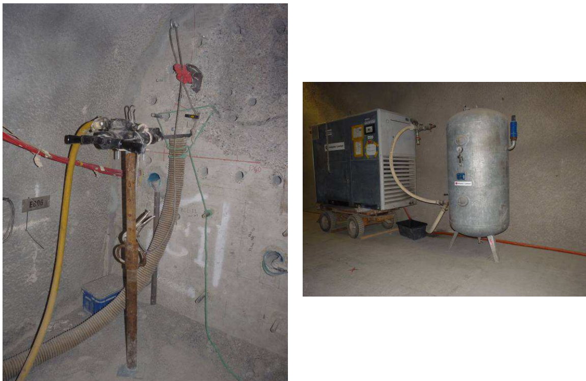
Figure 11: Pneumatic hammer and compressor (left/right)
