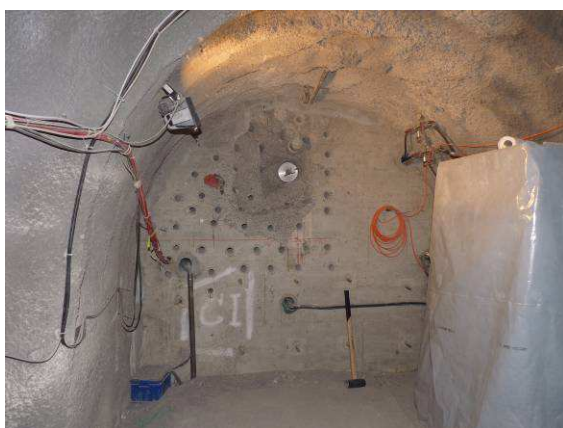
Holes around the main opening in the plug
