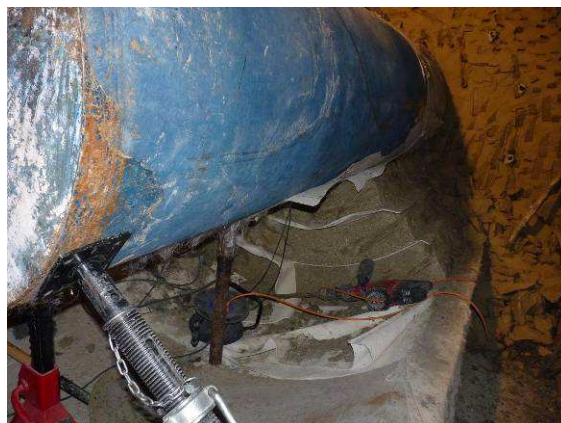
Temporary support of the canister
