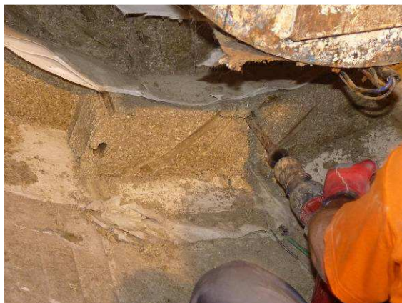
Figure 20: Tools for bentonite blocks removal
