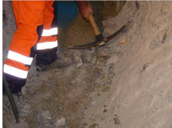
Use of hand tools to remove the concrete plug after the effect of the expansive cement (II)
