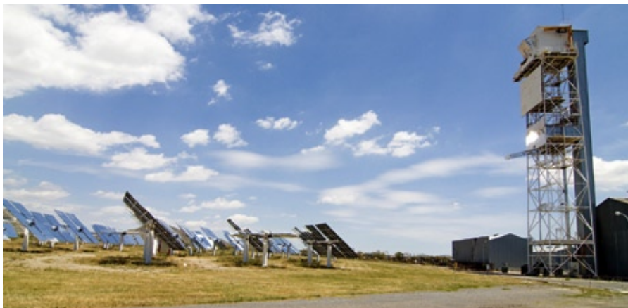
Vista general Hydrosol. General View of Hydrosol.
