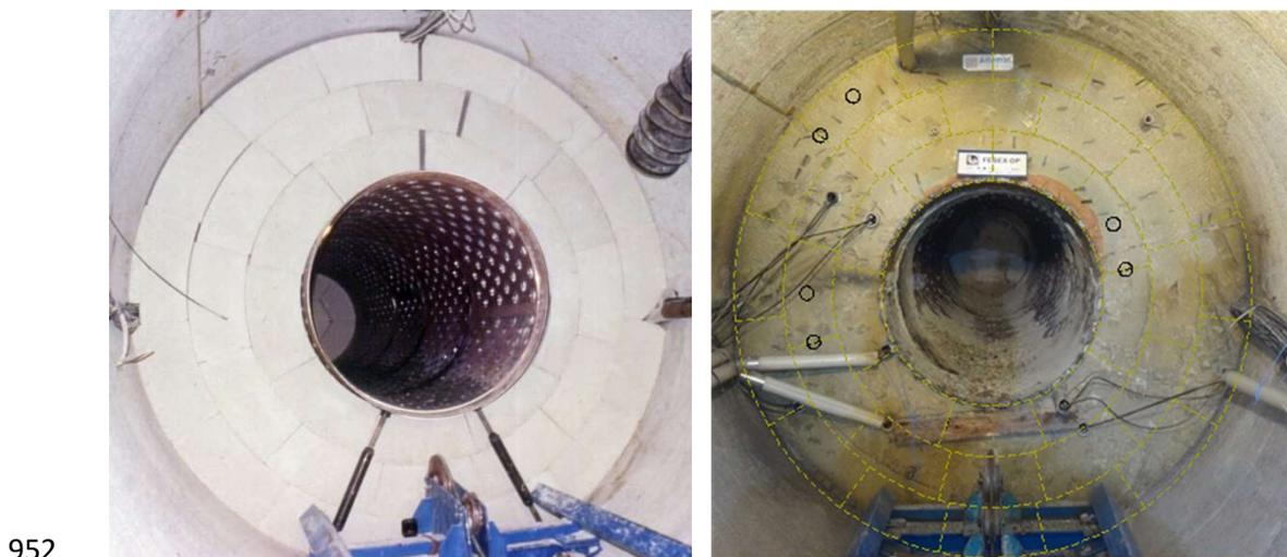
953 **Fig. 2:** Appearance of the bentonite barrier around Heater #2 during installation in 1997 and during
