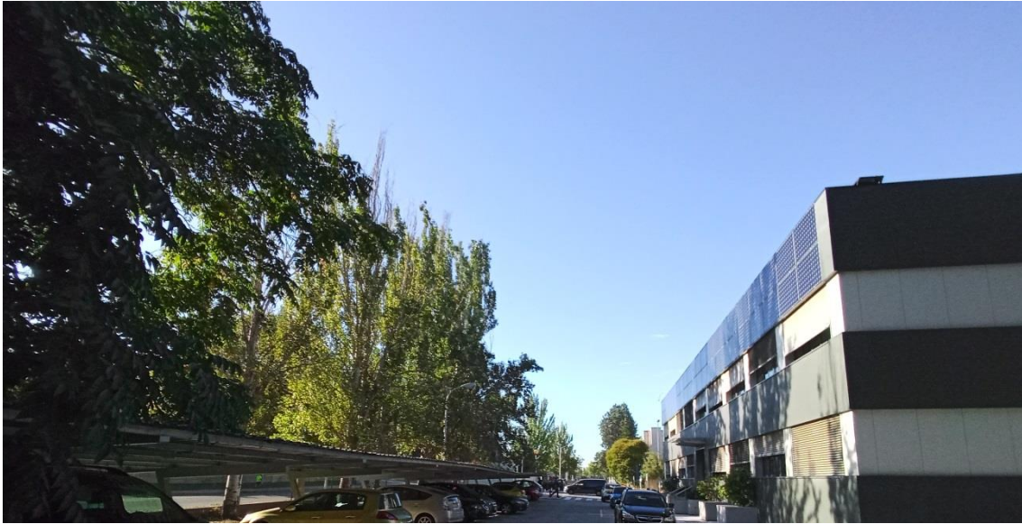
Figure 9. Irregular shading on the east facade caused by trees in a summer morning.
