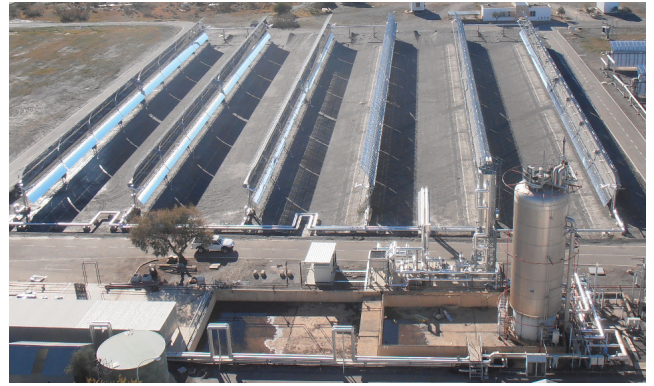
Fig. 3. Top view of the TCP-100 field at Plataforma Solar de Almería (PSA-CIEMAT). The three loops are shown, with two PTCs in each of them, numbered from 1 (rightmost) to 6 (leftmost). The first loop is formed by the connected pair 1-2 (right loop), the second loop by 3-4 (center loop) and the third by 5-6 (left loop).
