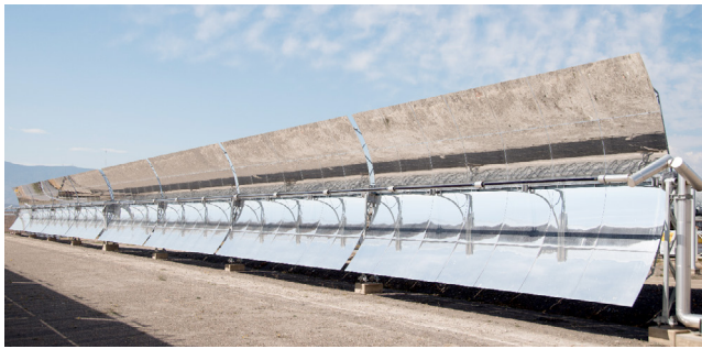
Fig. 2. Lateral view of the first TCP-100 PTC in the first loop at Plataforma Solar de Almería (PSA-CIEMAT). It is composed of 8 modules of 12 meters length.
