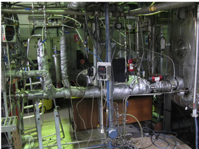
Fig. 2. Side view of the main injection line and the vessel.
