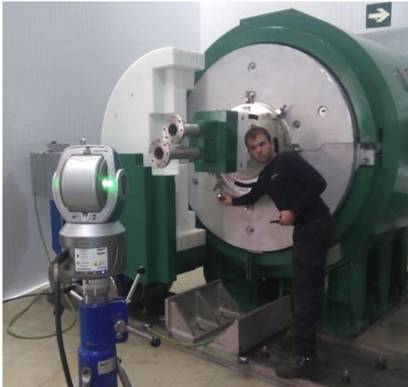
Figure 30 Realignment of the beam dump cartridge.
