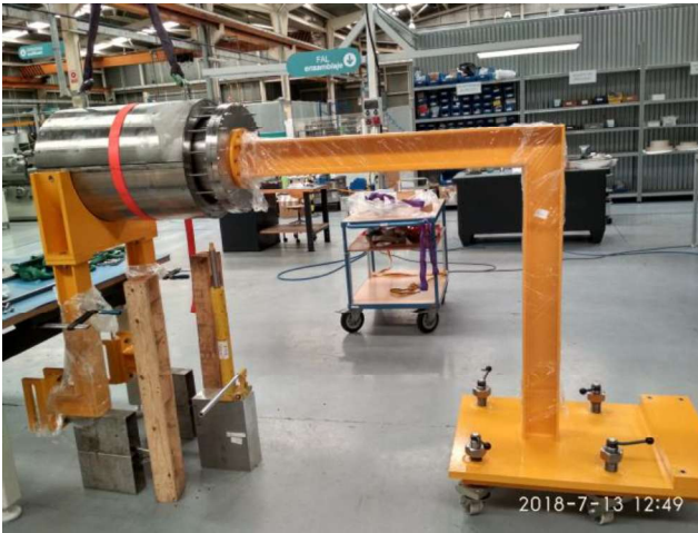
Figure 28: Temporal support structures for the installation of the conical tube through the beam dump cell wall. The yellow structure on the right will hold the conical tube from the inside of the beam dump cell. The yellow pieces on the left will be supported on the lead shutter support frame.
