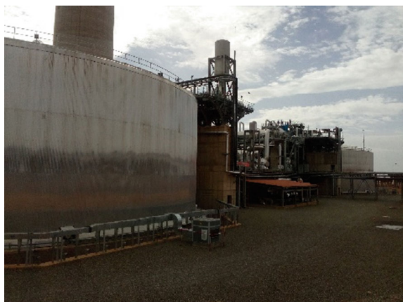
Fig. 1 Molten salt thermal storage system at MASEN (Morocco)
