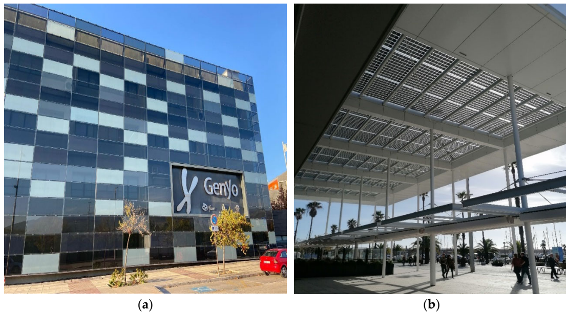
Figure 6. (a) BIPV double-skin façade in a research centre in Granada, Spain, with semi-transparent PV glazing in different tones (Onyx Solar, Avila Spain). Architects: E. Vallecillos and E. Rodríguez. Photo credits: Eva Ruiz. (b) Photovoltaic pergola with crystalline silicon glazing having 18% light transmittance (Onyx Solar) at the Olympic Port in Barcelona, Spain. Photo credits: Carmen Martín.
