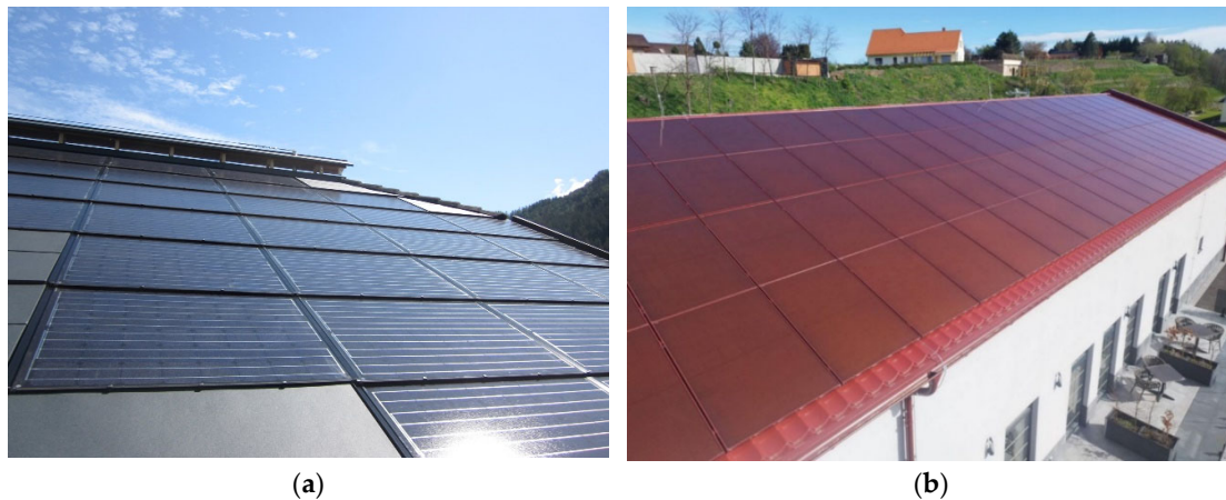
Figure 4. (a) Innovative BIPV solution for a roof in Badia, Italy. BIPV modules and mounting system (Solar-Fabrik, Laufach, Germany, and Ernst Schweizer AG, Hedingen, Switzerland) ensure a watertight seal. Source: GSE (GSE, 2012). (b) BIPV roof in a commercial building in Valtice, Czech Republic, with crystalline silicon terracotta-colour modules (Yingli Gain Solar, Baoding, China) to fit the urban context. Photo credits: Millie Tan.
