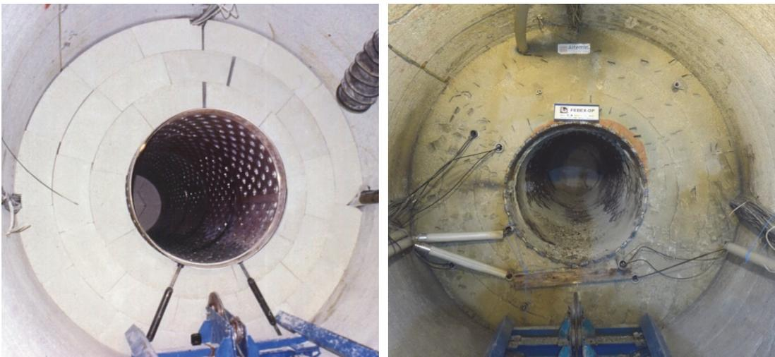
**Fig. 2: Appearance of the bentonite barrier around Heater #2 during installation in 1997 and during dismantling in 2015**
