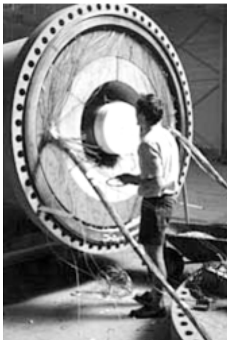
Figure 5. View of the PRACLAY Project mock-up before installation of the cover.
