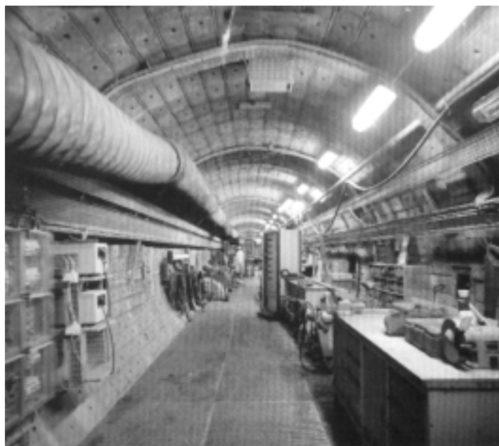
Figure 4. The HADES underground facility (Mol).
