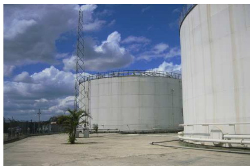
Illustration 7: Digesters of the vinasse treatment plant of Brugal
