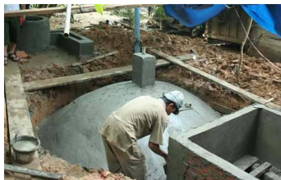
Illustration 1: Fixed-Dome Anaerobic Digester
