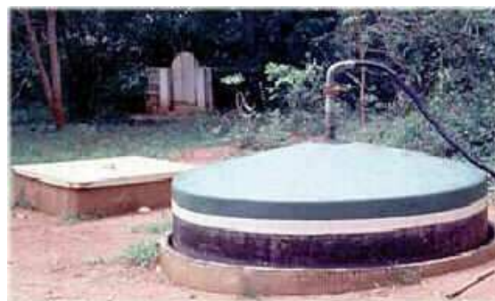
Illustration 2: Floating Drum Anaerobic Digester
