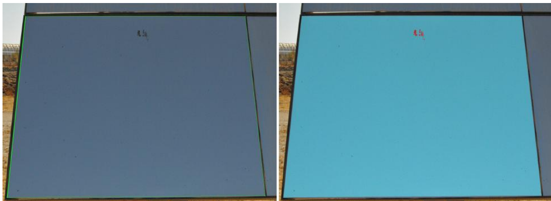
Figure 6. Images of one heliostat facet with well-defined corrosion: left) original image, right) after analysis, corroded area marked in red.
