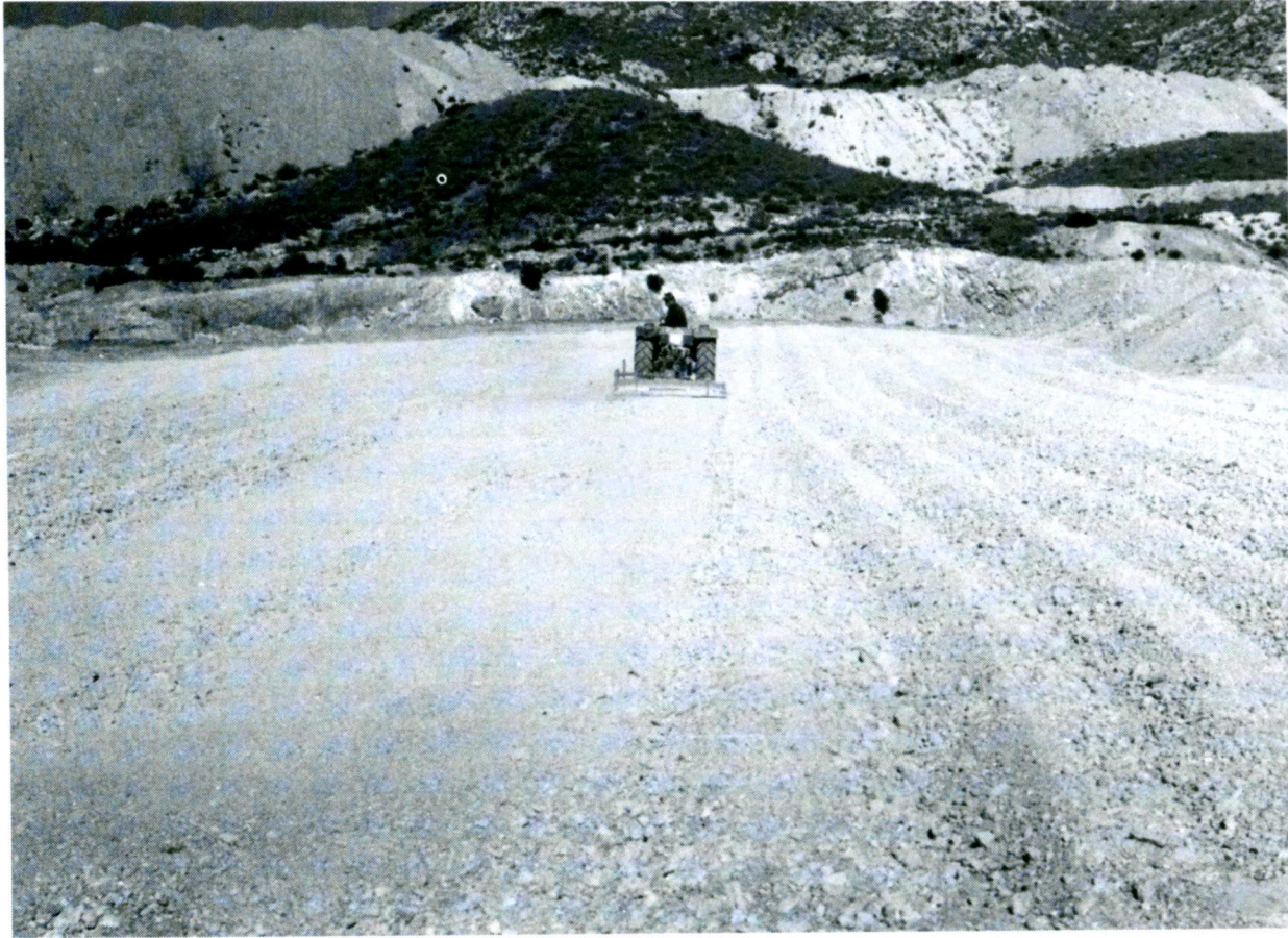
Figure 3.3: View of the conditioning site after a pass of the rotary cultivator.
