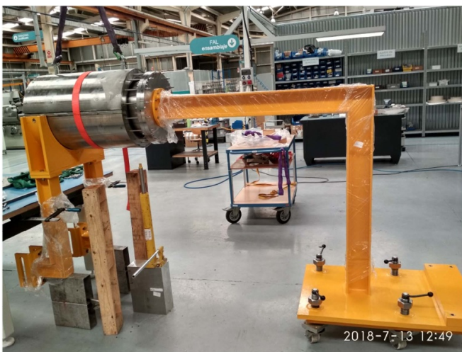
Figure 28. Temporal support structures for the installation of the conical tube through the beam dump cell wall. The yellow structure on the right will hold the conical tube from the inside of the beam dump cell. The yellow pieces on the left will be supported on the lead shutter support frame.
